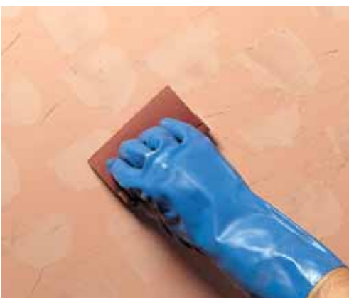
"Veneziano" effect: sand-papering between different coats of Silexcolor Marmorino with a fine grained abrasive sand paper
