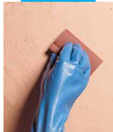
"Encausto" effect: sand-papering of Silexcolor Marmorino with a fine grained abrasive sand paper
