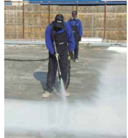
Application of Purtop 600 on a flat roof by spray
