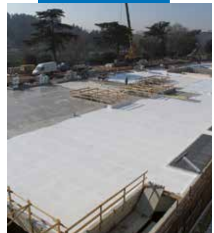
Covering of an underground car-park waterproofed with Purtop 600
