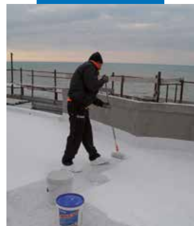
Application by roller of Triblock P on a concrete surface
