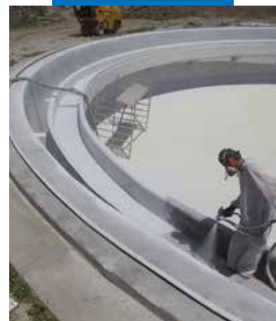
Application of Purtop 1000 onto industrial storage tanks
