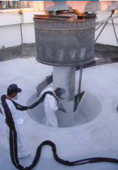
Particulars of a Purtop 1000 waterproof coating applied on various substrates (cementitious and metallic)
