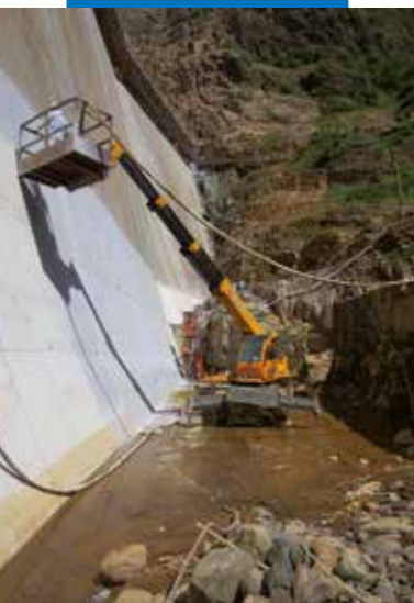
Waterproof coating on a dam
