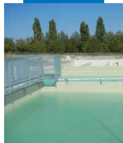
Storage tanks waterproofed with Purtop 1000
