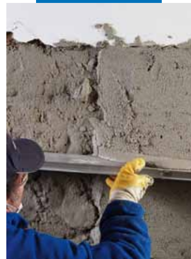
Levelling PoroMap Intonaco with a straight-edge
