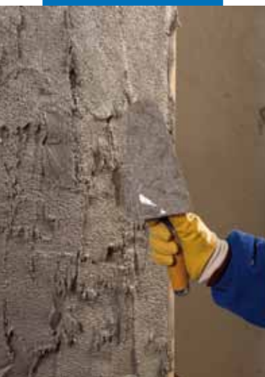
Application of PoroMap Intonaco by trowel
