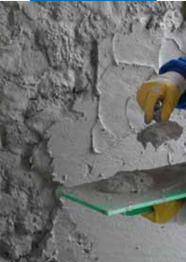
Application of PoroMap Intonaco by trowel
