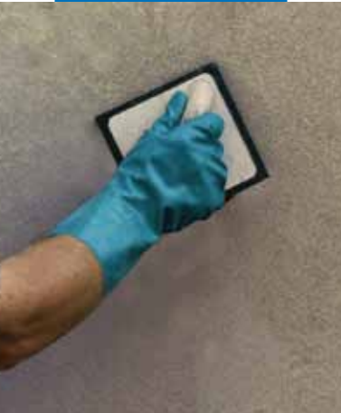
Finishing off the surface of PoroMap Finitura with a sponge float
