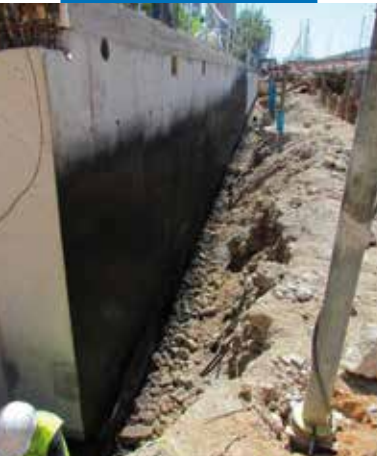
Foundation wall waterproofed with Plastimul 2K Reactive
