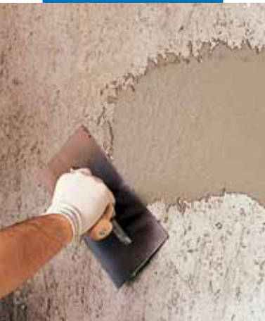
Applying Planitop 540 with a metal trowel
