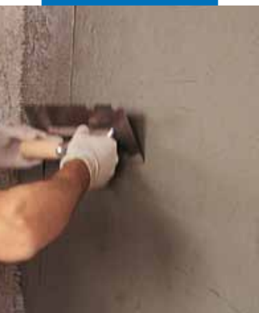
Applying Planitop 540 with a metal trowel
