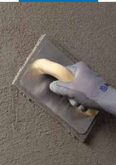
Floating the surface of Planitop 517
