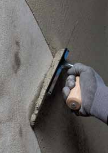
Application of Planitop 517
