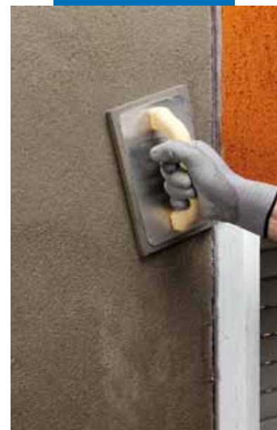
Floating the surface of Planitop 217
