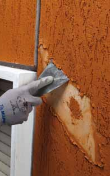
Removing all the plastic covering that has not adhered
