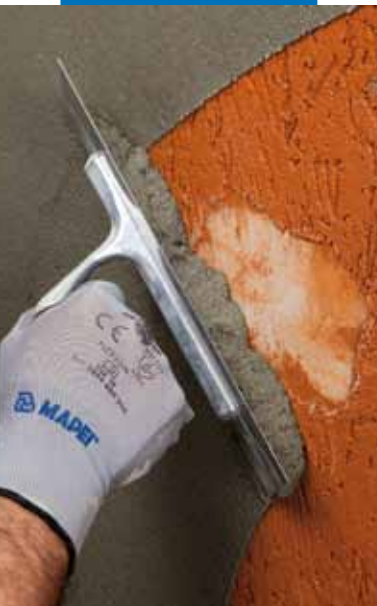
Application of Planitop 217
