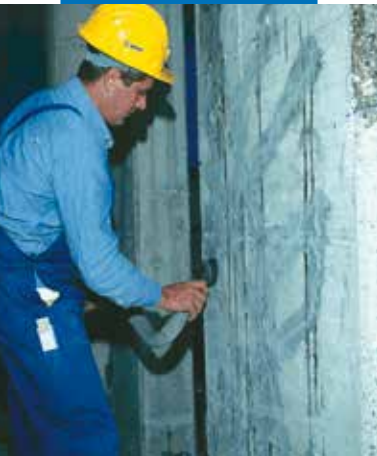
Preparing the substrate
