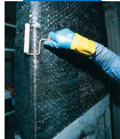
Applying a second coat of MapeWrap 31
