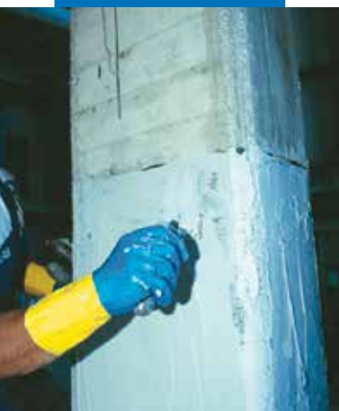
Smoothing with MapeWrap 11 or MapeWrap 12
