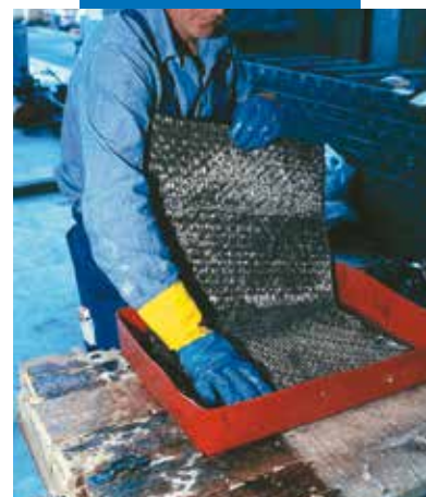
Manually impregnating MapeWrap C
