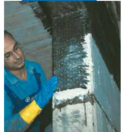
Wrapping columns and beams
