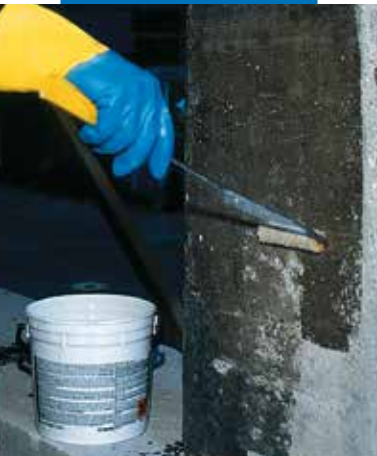
Applying MapeWrap 31 with a roller on the still fresh MapeWrap 11 (or MapeWrap 12)
