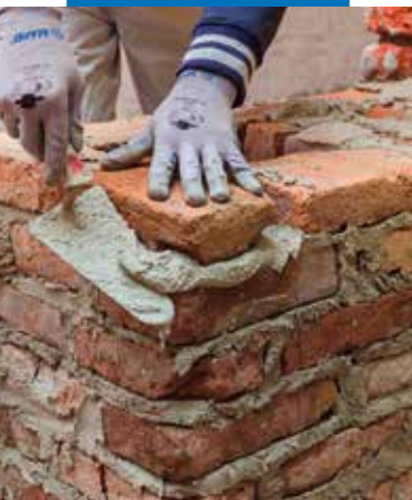
Forming the installation bed
