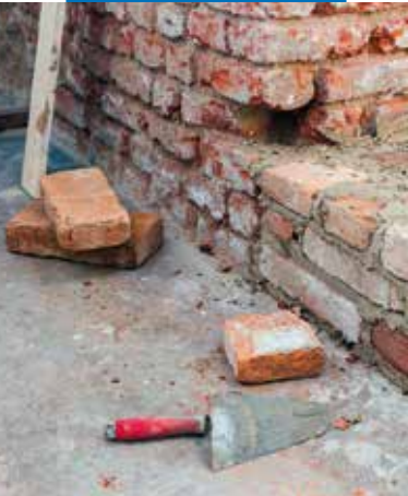
Re-building a masonry
