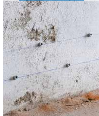
Detail of the staggered rows of holes
