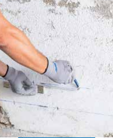
Preparing the holes
