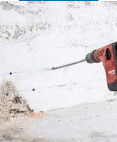
Drilling the holes
