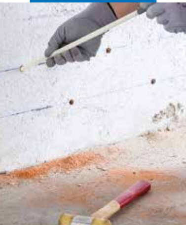
Inserting the injectors in the holes
