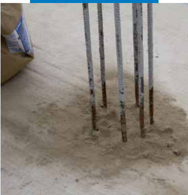
Application of Mapeproof Seal before a piece of Mapeproof bentonite sheet
