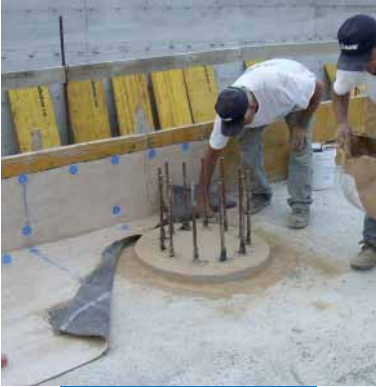
Application of Mapeproof Seal around a pile head
