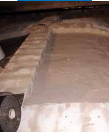
Application of the first layer of Planitop HDM Restauoro
