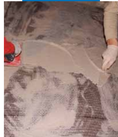
Application of the second layer of Planitop HDM Restauro
