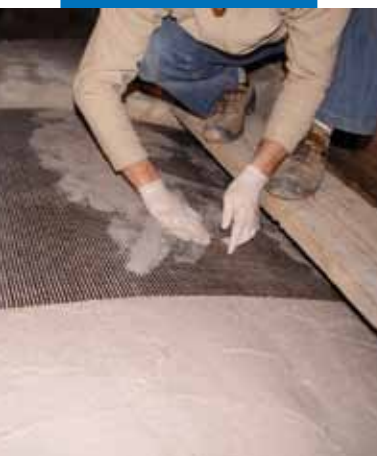
Positioning of Mapegrid B 250
