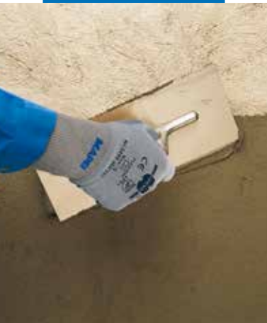
Application with trowel
