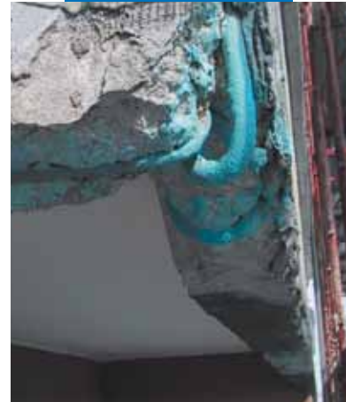
Reinforcing rods on the front side of a balcony treated with Mapefer 1K
