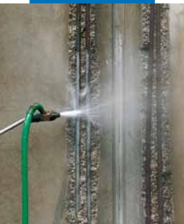
Cleaning reinforcing rods
