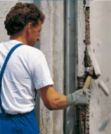
Demolition of degraded concrete
