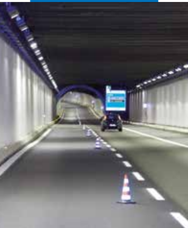
Support walls treated with Mapecoat I 650 WT
