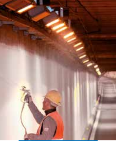
Application of Mapecoat I 650 WT
