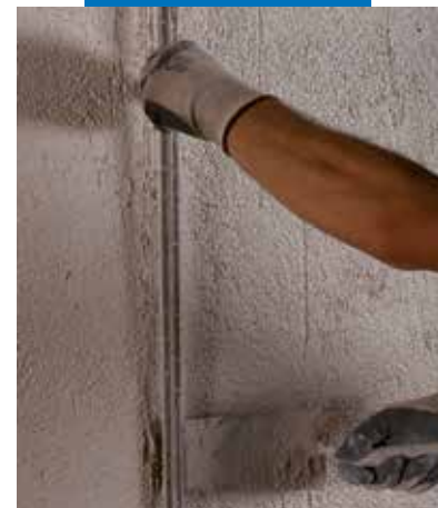
Removal of the vertical guide
