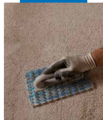
Planing the surface of Mape-Antique MC Macchina
