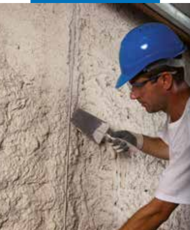
Positioning a vertical guide
