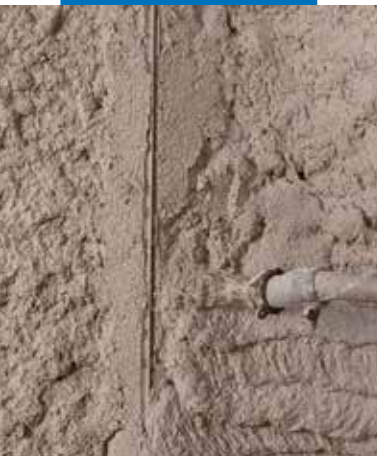
Application of Mape-Antique MC Macchina
