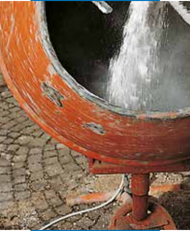
Mixing mortar on site with locally-sourced aggregates
