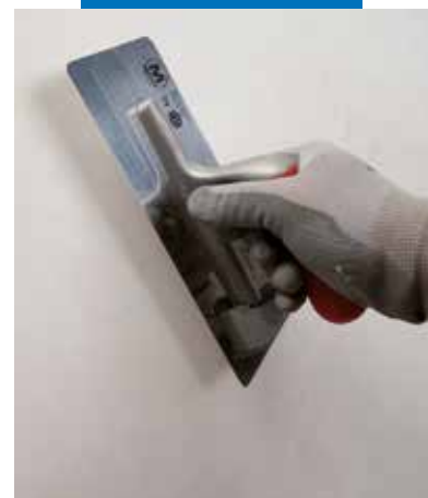
Spread on a second layer of Mape-Antique FC Ultrafine
