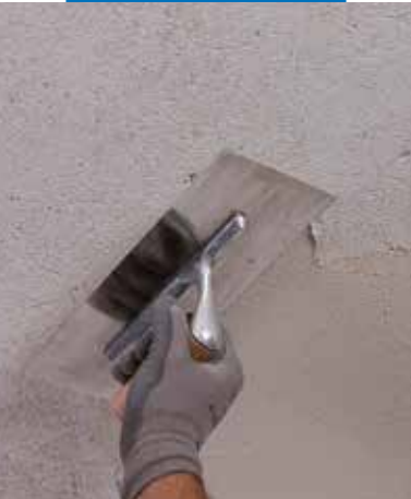
Application of Mape-Antique FC Grosso
