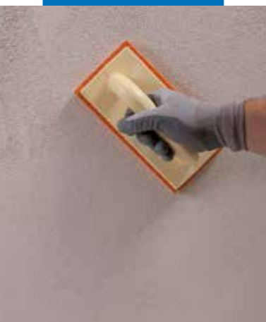
Finishing the surface of Mape-Antique FC Grosso with a sponge float
