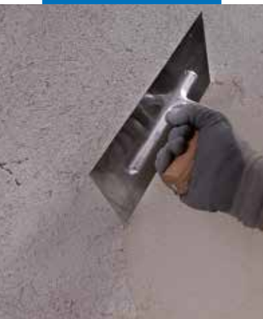
Application of Mape-Antique FC Grosso
