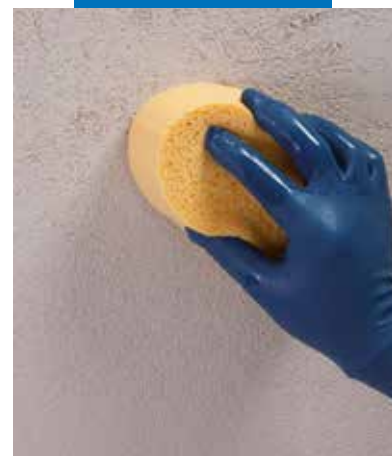
Finishing the surface of Mape-Antique FC Grosso with a sponge
