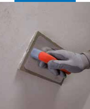
Finishing with a damp sponge float of Mape-Antique FC Civile
