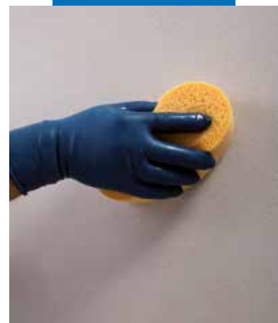
Finishing the surface of Mape-Antique FC Civile with a sponge
