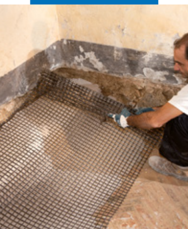
Positioning Mapegrid G 220 alkali-resistant glass fibre reinforcement mesh
