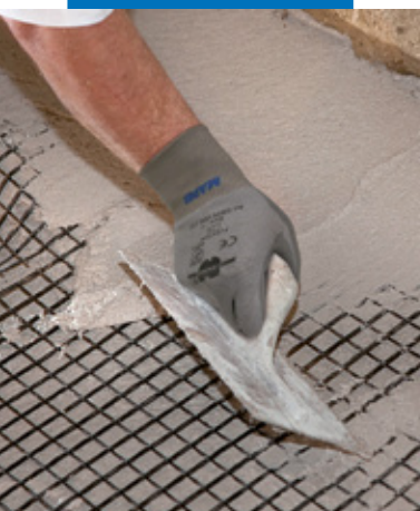
Application of the second layer of Planitop HDM Restauro by trowel on the outer face of a vaulted ceiling to cover the Mapegrid G 220 with an even coat
