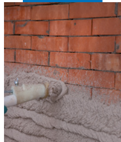
Application of Planitop HDM Restauro by spray on a brick wall
