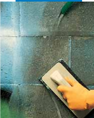
Cleaning with an abrasive pad
