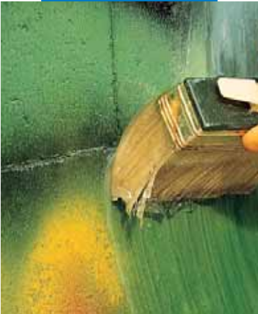
Applying WallGard Graffiti Remover Gel with a brush
