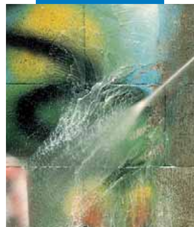
Using a high-pressure cleaner
