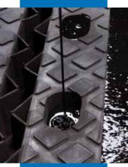
Casting neat Mapeflex PU65 into the anchorage points
