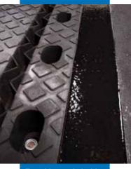
Transition sealed with Mapeflex PU65 mixed with sand
