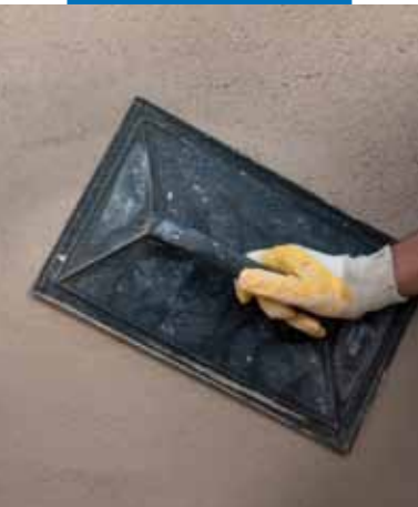
Levelling the render
