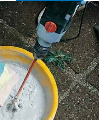
Preparation of Mape-Antique I
