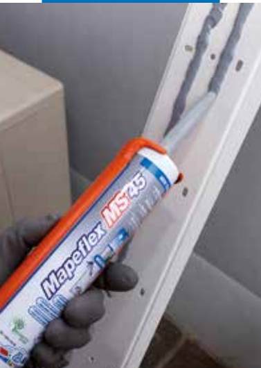
Bonding plastic profiles on a surface outside
