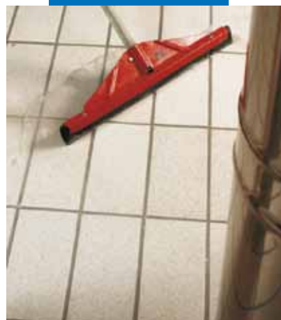
Cleaning off the flooring surface with a rubber raker
