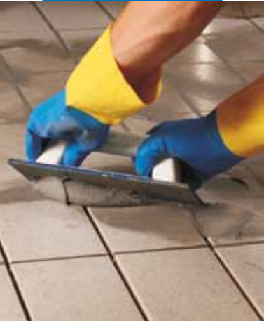
Grouting floor joints with a rubber trowel
