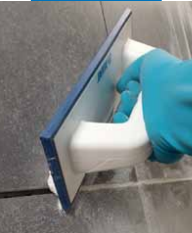
Laying Flexcolor with a rubber trowel
