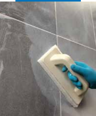
Cleaning the joints with a Scotch-Brite® pad
