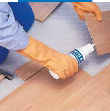
Applying Adesivil D3 to the grooved section of laminate flooring
