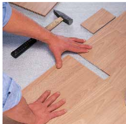
Placing tongue-and-groove sections of laminate flooring
