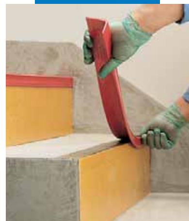
Installation of a PVC step nosing
