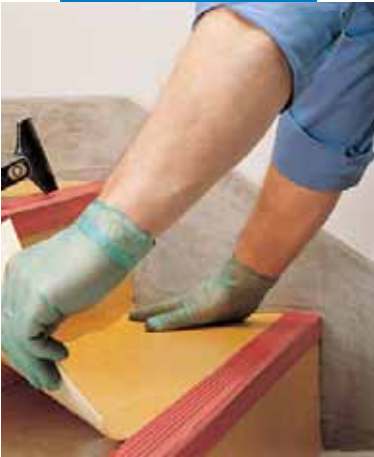
Spreading Adesilex VZ of the backing of a PVC covering
