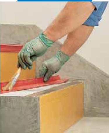
PVC installation on a step
