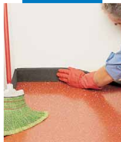
Bonding of PVC skirtings
