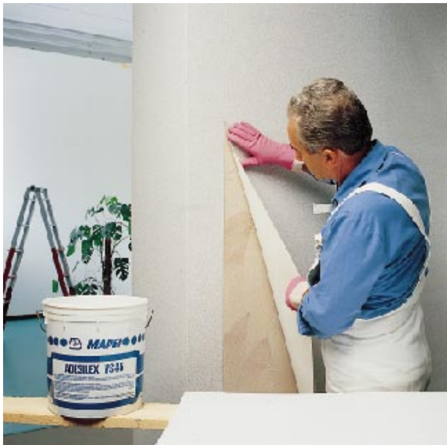
Applying ADESILEX VS45 with n. 1 trowel
