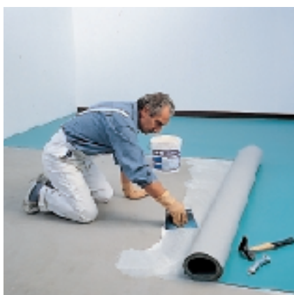
Homogeneous PVC sheets being installed over ADESILEX V4
