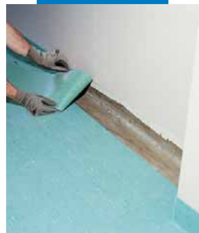
Installing PVCA flanking strip
