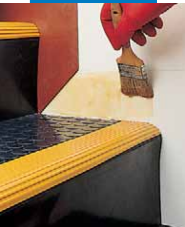
Installing rubber skirting with Adesilex LP
