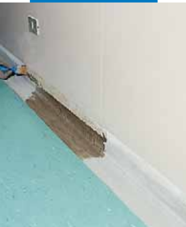
Installing Liuni PVC flanking strip with Adesilex LP
