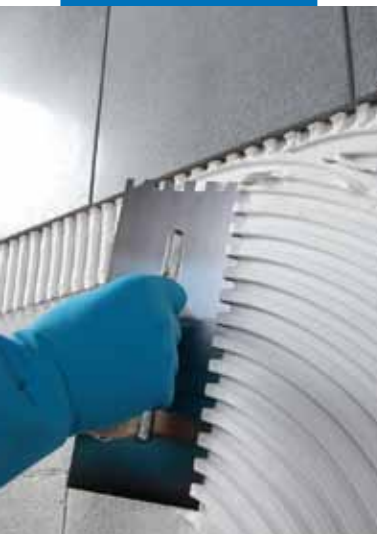
Spreading Ultramastic 5 on a substrate
