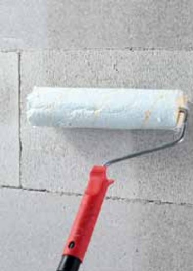
Application of primer on a substrate made from lightweight concrete blocks
