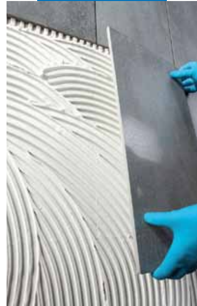
Fixing large-sized tiles on lightweight concrete blocks
